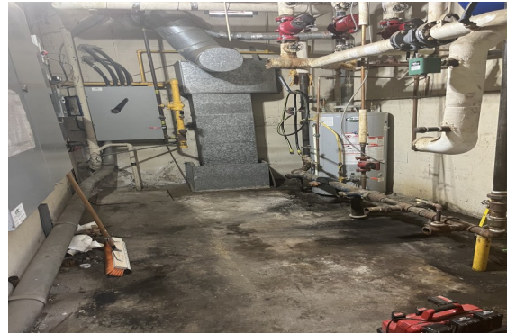
Empty Room after Demolition and Removal
